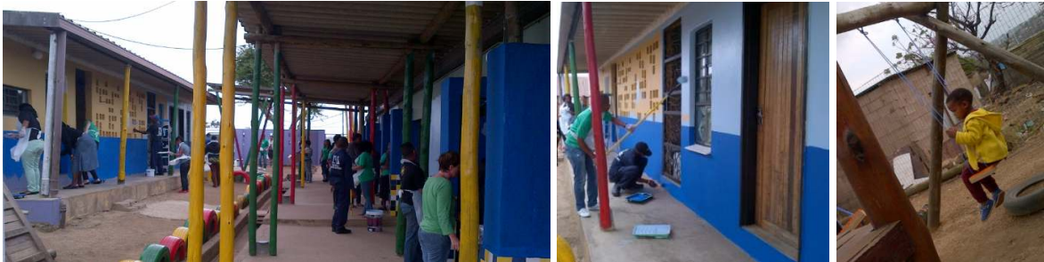
September 2014 - painting, swing repair and other work at Kulakahle Crèche
